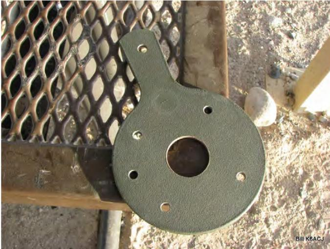
Guy Ring and Lanyard Support Ring Detail. The hole pattern is for either 3 guy ropes or 4 guy ropes. Chamfer the holes to prevent chafing the ropes.
