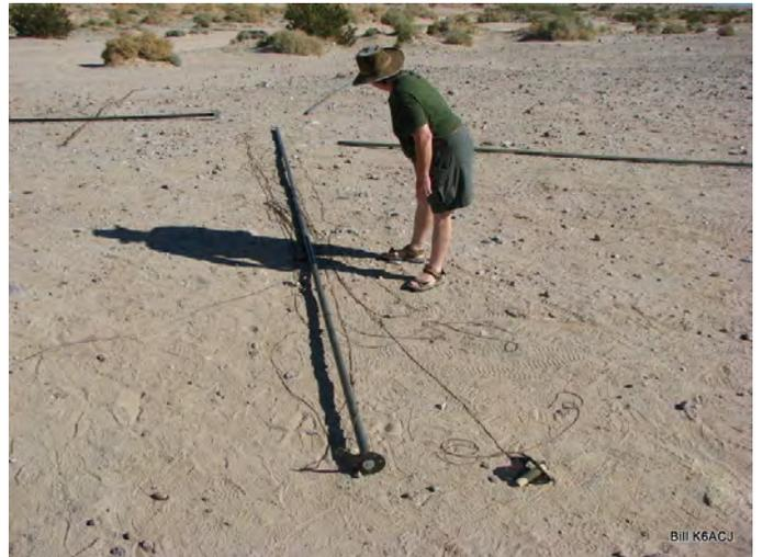
Peter VE7REZ/W6 is shown measuring the mounting position for each of four masts and measuring the final cut on the guy ropes down from the top of each mast. Each mast is supported at the bottom in a hole in the ground roughly 10 inches deep then with one person on each of the 3 guy lines the mast is pulled up into position and staked down. Expect the desert floor to be rock hard but the advantage is that it firmly holds the mast and ground stakes.
