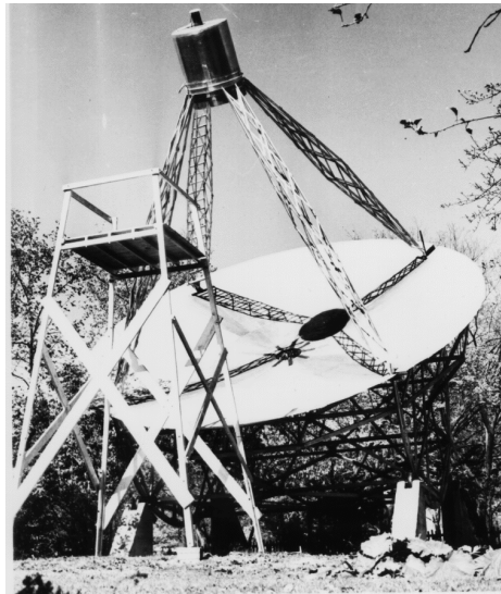
Grote Reber's original antenna constructed in his back yard in Wheaton Ill about 1937.
