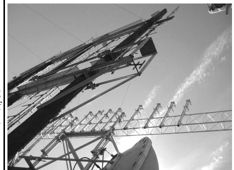
Empty antenna mounts at new site.
