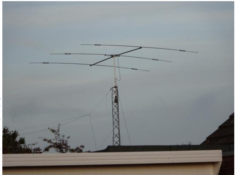
A tri-band beam antenna spotted by Spencer in England. He's always on the lookout for ham antennas!
