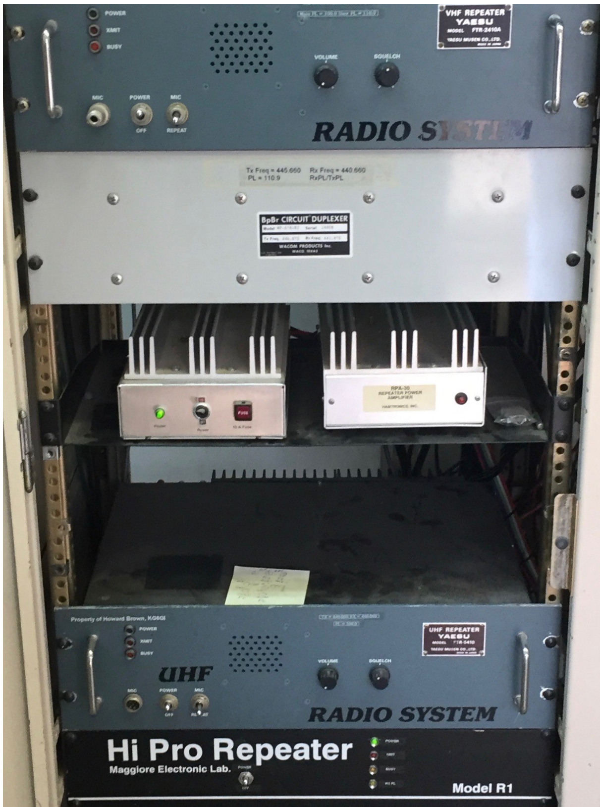
From Top: FTR-2410 2 Meter Repeater, VHF & UHF Power Amplifiers, FTR-5410 UHF repeater, Maggiore 220 Repeater
