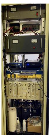
At the SOARA San Clemente repeater site, the ACC RC-850 repeater controller has been replaced with an Audio Test Solutions (Formerly Link Communications) RLC-4 controller. By standardizing on RLC controllers, we have simplified our ongoing maintenance. The common platform will also allow us to standardize repeater commands for our users.
