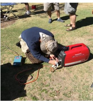
Jim, KI6LOM grounding the generator to reduce significant noise. The noise was driving Ray AE6H crazy until we grounded the generator. It was an amazing demo with Jim's scrap wire and a screwdriver ground rod. Jim is good at improvising!
