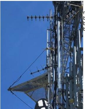
This is the old location on the Yagi pole WR6AAC repeater antenna is second from bottom with a bent boom. The SOARA antenna is the 3<sup>rd</sup> one from the bottom and elements are twisted, later ice hit it and bent boom also.
