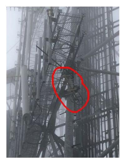
The new location under the cross arm, it's hard to see as we were in the clouds that day and it was windy and cold! So, if you look closely the SOARA antenna is gold on the bottom and is horizontally polarized. The black WR6AAC antenna is directly above and vertically polarized.
