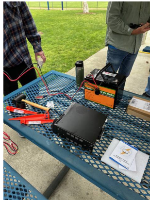
Large battery demo
